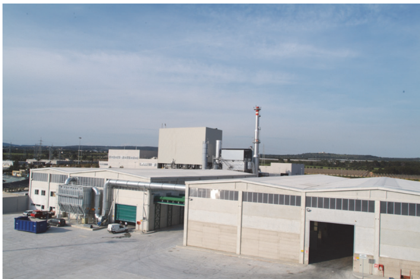
Photo 1. General view of the Massafra plant
