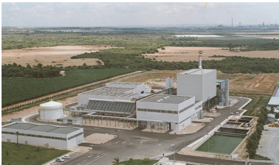
Photo 5. General view of the power station for energy recovery
