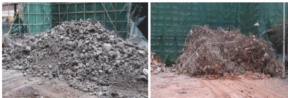
Fig. 9. Sorted broken concrete and steel stockpiled separately (Public Fill Committee, 2004)
