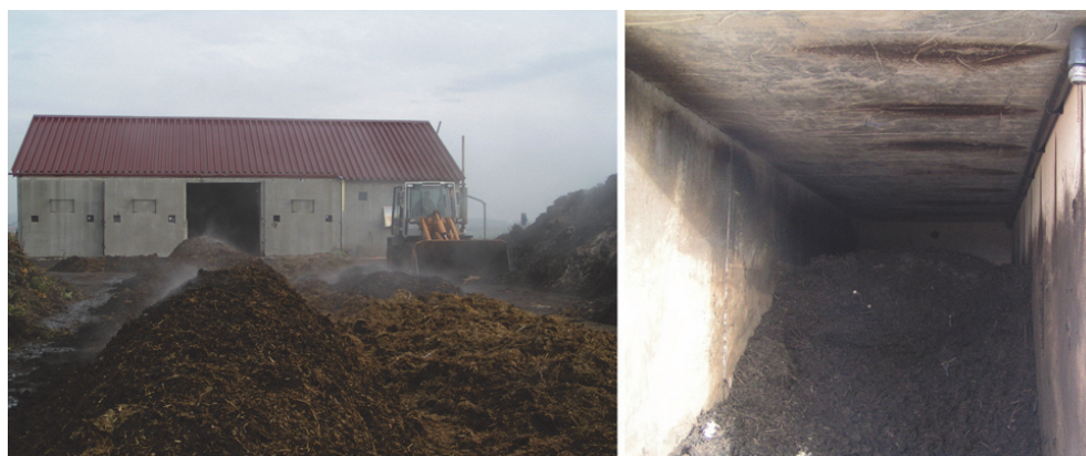
Fig. 3. Full-scale farm plant with four solid-phase digestion boxes
