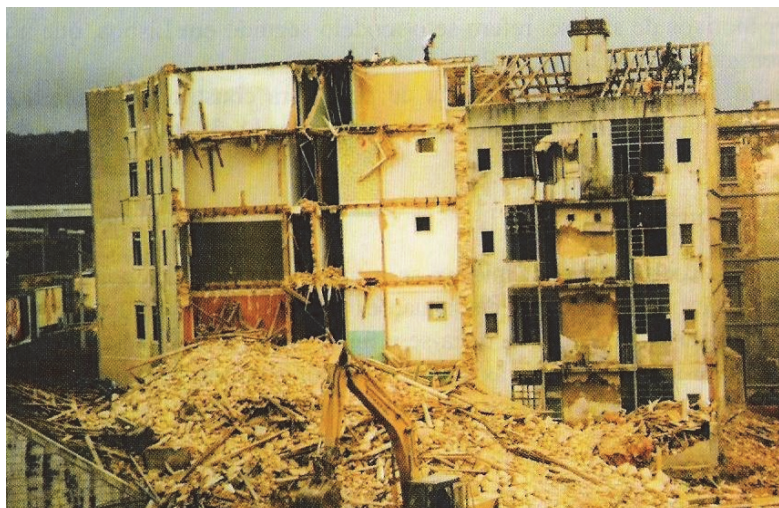
Fig. 8. Sample of an undifferentiated demolition. Source: (Pinto, 2000)
